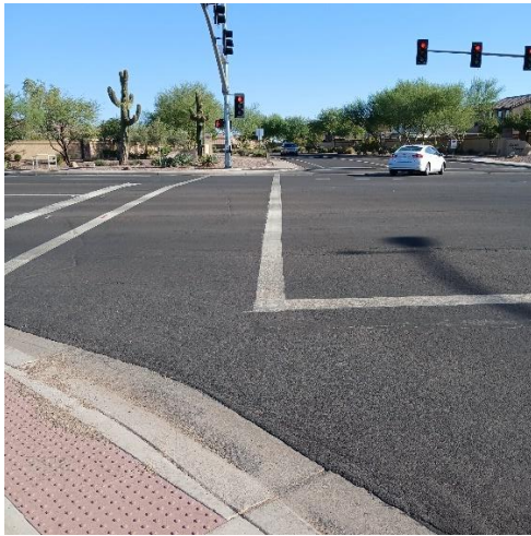
S W corner of W. Bollin Rd and Smith Farms Circle facing north. Descriptive of incorrect crosswalk markings, high visible yellow would cover curb to curb.
