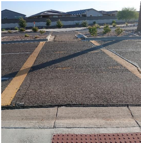
Crosswalk on SW Honeycutt facing N E just before entering roundabout, incorrect markings and degraded median needing repair.
