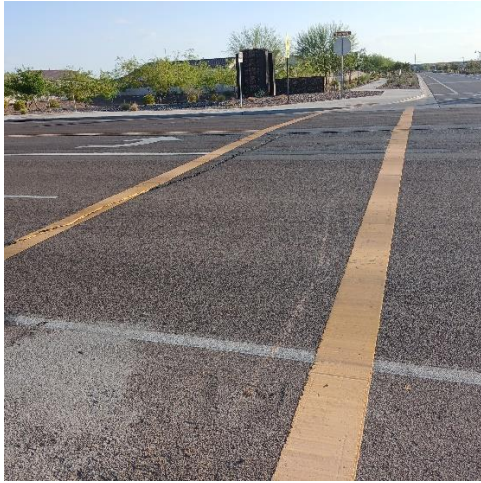
School crosswalk on SW Honeycutt Rd and E. Costa Del Sol Blvd. facing N E within 600 feet of school driveway. Incorrect markings for school crosswalk.
