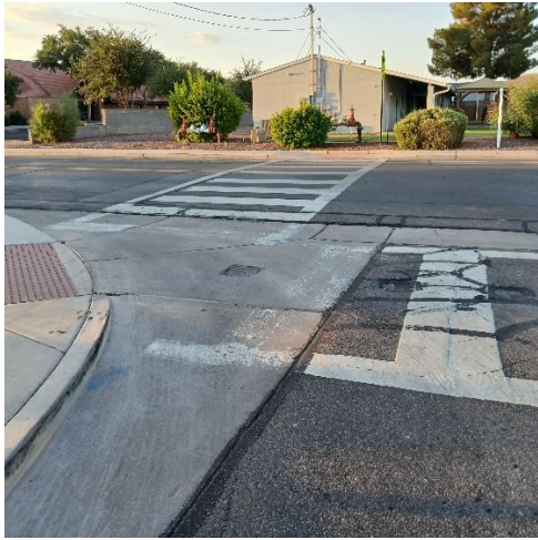
N E corner of Taft Avenue and W. Honeycutt facing south depicting incorrect and degraded markings.
