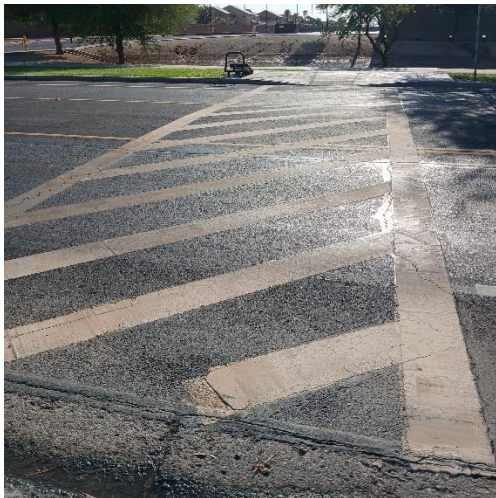
Crosswalk on North Casa Del Sol Blvd facing E. The crosswalk is marked correctly but is degrading.
