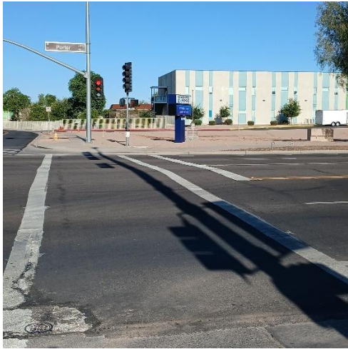
N E corner of Porter Rd at Adams facing west towards Leading Edge Academy. School crosswalk is incorrectly marked at a four-way controlled intersection.
