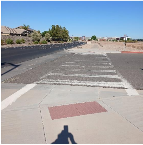
Crosswalk at S W corner of school driveway and W. Allen Stephens Pkwy facing east. Crosswalk is incorrect color, no school crossing sign, and no stop line.
