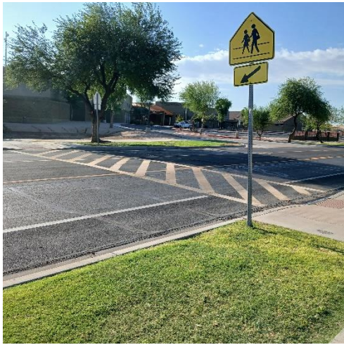
Crosswalk on North Casa Del Sol Blvd facing S E towards the school. The crosswalk is marked correctly but is degrading.
