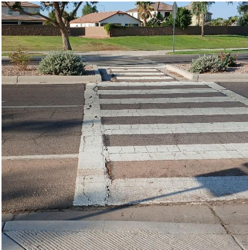
Crossing at the roundabout on Honeycutt and North Casa Del Sol Blvd facing S W. Crosswalk is incorrect markings and degraded, not ADA compliant.
