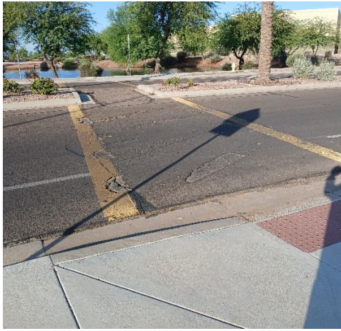
Degraded crosswalk exiting S W round about. Incorrect markings and not ADA compliant.
