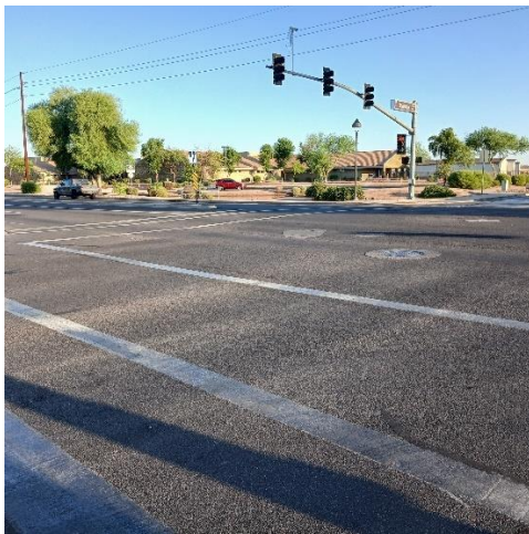
Incorrectly marked school crosswalk on W. Honeycutt and North Donithan Rd. at S E corner facing N W.
