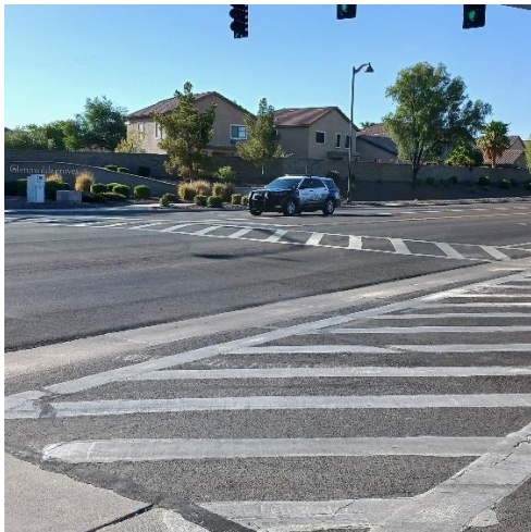
N W corner of Porter Road and Adams facing S E depicting incorrect School crosswalk markings.
