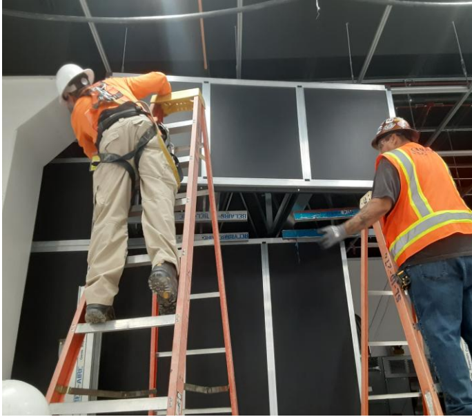
Follett: Assembling the head piece to a CRAH unit inside a data hall at CyrusOne Chandler, Arizona.
